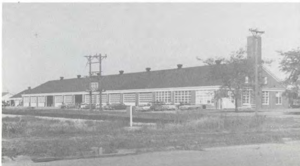
Shown here is the south side of the Navy Transportation Shop, which became the Furnas Building on CNTCC. The 31,578 square foot building was equipped with automotive pits and a paintshop. Many hand tools and other equipment items were left by the Navy and utilized by the college.
