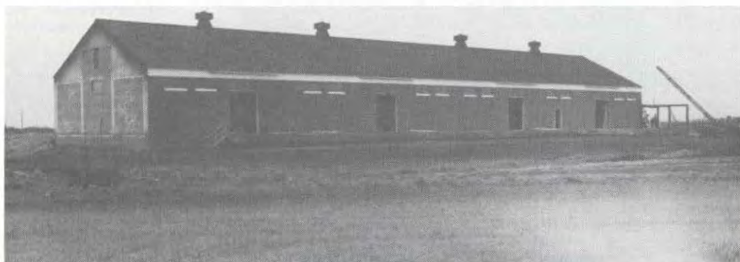
This building, to be known as the Webster Building, was to be the location of the agricultural-related programs. Renovation of the building began in 1969, and included covering the loading dock to gain additional usable space.
