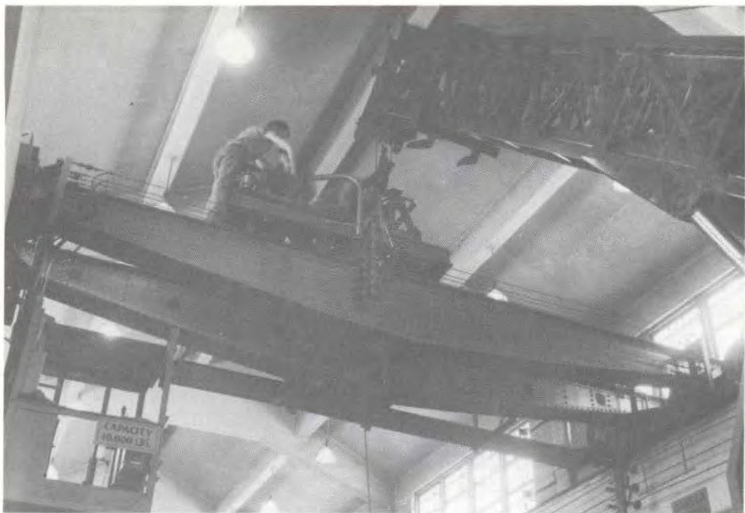
In March of 1970 work began to dismantle and remove the 5 ton overhead electric crane from the Hamilton Building. The college having no use for the traveling crane had sold the unit.
