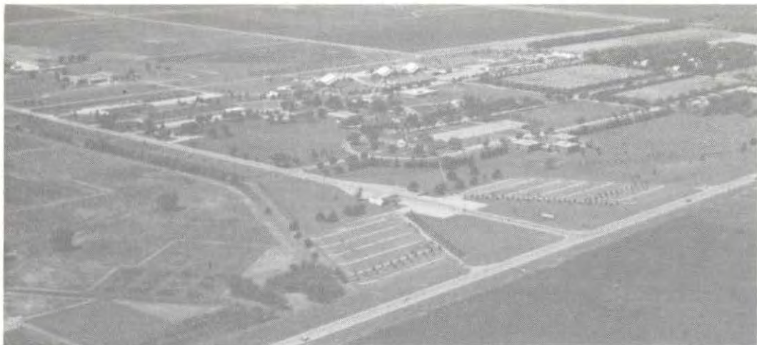
The Hastings Campus as it appears in 1984. Many things have occurred since the college assumed the facilities in 1966.
