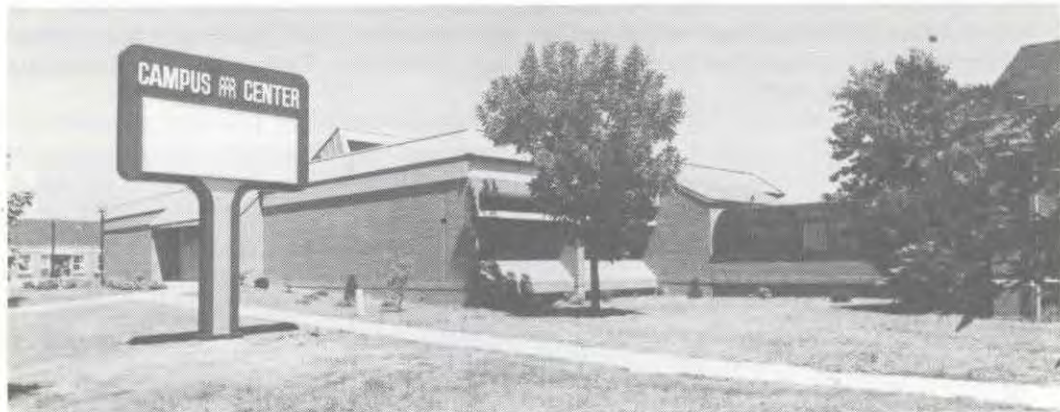
The Campus Center after completion, the facility has become the center of student activity and regularly serves as the focal point for activities conducted on the Hastings Campus.
