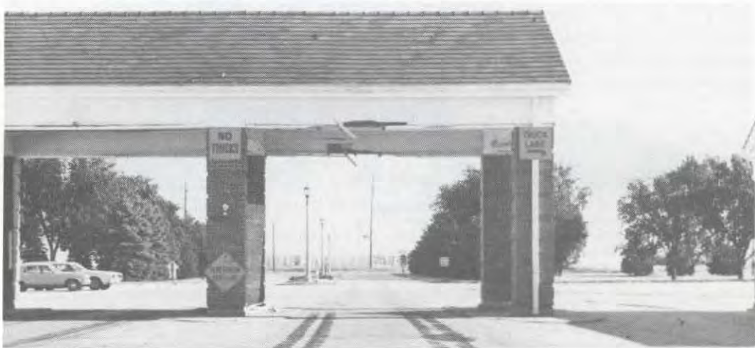
For a number of years this was a common scene at the main gate to the campus. The college finally removed the canopy at the main entrance.
