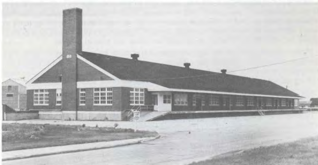
The Navy Supply Building (Building #13) as it appeared in 1966. At the time CNTC occupied the site, this building was under the control of the U.S. Army Corps of Engineers being used by the U.S. Army Reserve. This building would eventually be occupied by the college and later named the Nuckolls Lab.
