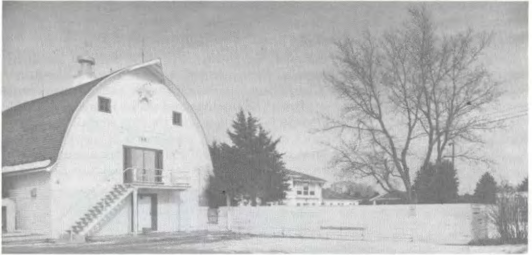
Building #48, the former Air Force Officers' Club, was acquired by the college in 1968. The facility was renamed the Greeley Recreation Building by the college.
