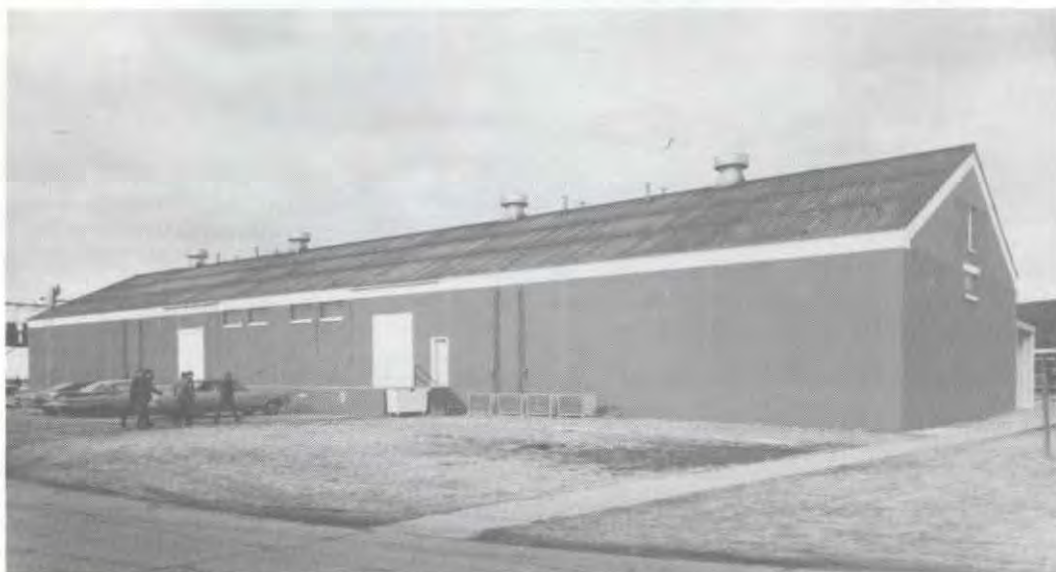
The Kearney Laboratory was renovated in 1969 and 1970. The electronics program was located in the facility and remains there today.
