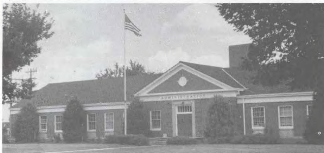
Top, the Navy Dispensary under construction in 1943. Bottom, the same building in 1966 after the college took possession of the facilities. The building has continued to serve as the campus administration building since 1966.
