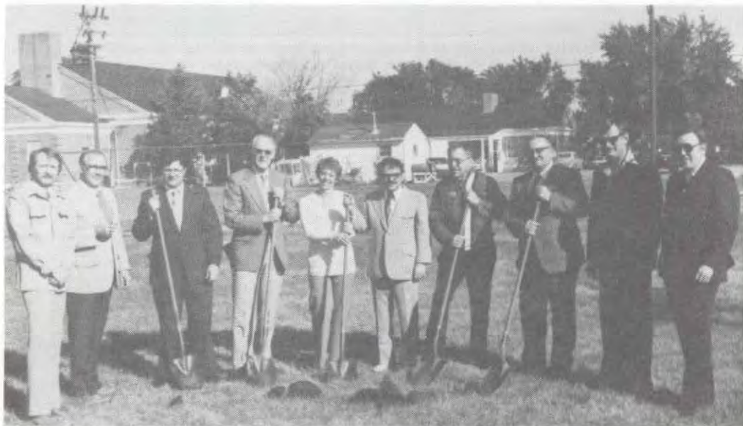
Construction of a health occupations building on the Hastings campus was approved in 1976 by the Board of Governors. Several months later groundbreaking was held. From left: Hal Friborg, architect; Ed Minnick, Dean of Students; Dennis Tyson, Dean of Instruction; Dr. Chester H. Gausman, Area President; Kathleen Mast (McPherson), Health Cluster Chairperson; Dr. Michael Paradise, Hastings Campus President; Ken Wortman, and Irv Schwartz, Board of Governors members; Vince Krueger, Director Physical Plant; and Don Nispel, architect.
