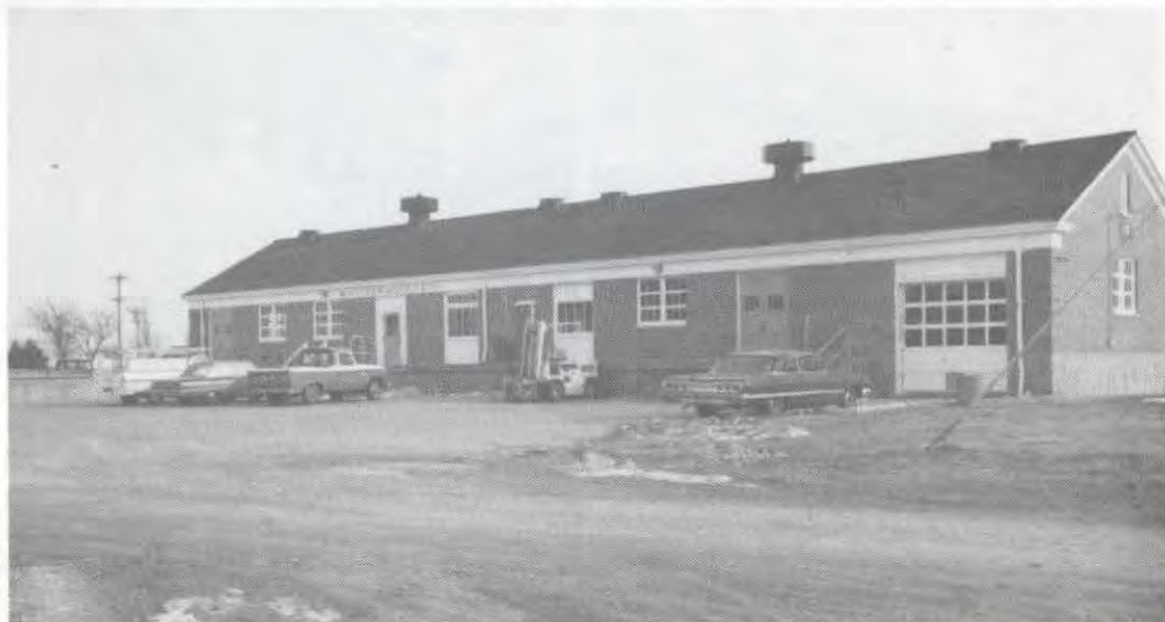
Building 15, later to become the Howard Building, served for a number of years as the headquarters for the campus maintenance department. The photograph above was taken in January 1970. Later that year, the building was renovated for use as an instructional facility.
